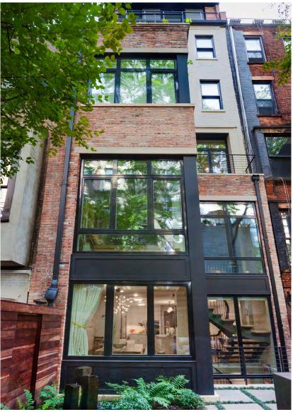
THE EXISTING PAINTED REAR **BRICK FACADE** WAS STRIPPED, **RESTORED AND EXPANDED WITH CORNER OPENINGS** AND A NEW ADDITION.
