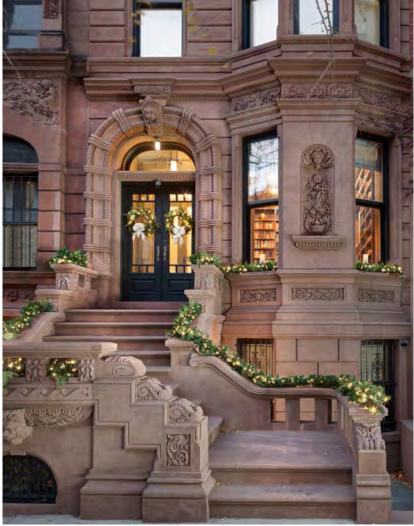
**BEFORE AFTER**  **FACADE THAT WAS REMOVED IN** THE 1940'S WAS REINSTALLED, ALONG WITH A **NEW STOOP MATCHING THE NEIGHBORING BUILDINGS IN THE** SAME ROW. THIS WAS POSSIBLE BY **INSTALLING ALL PASSIVE DETAILS** ON THE INTERIOR.
