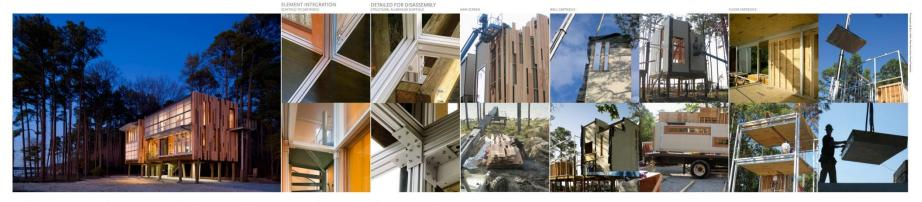
Loblolly House, located on the shore of the Chesapeake Bay, represents a novel approach to pre-fabricated and modular housing concepts. The house introduces off-site fabricated elements which are detailed for on-site assembly, future disassembly and redeployment. diversion design intent.
